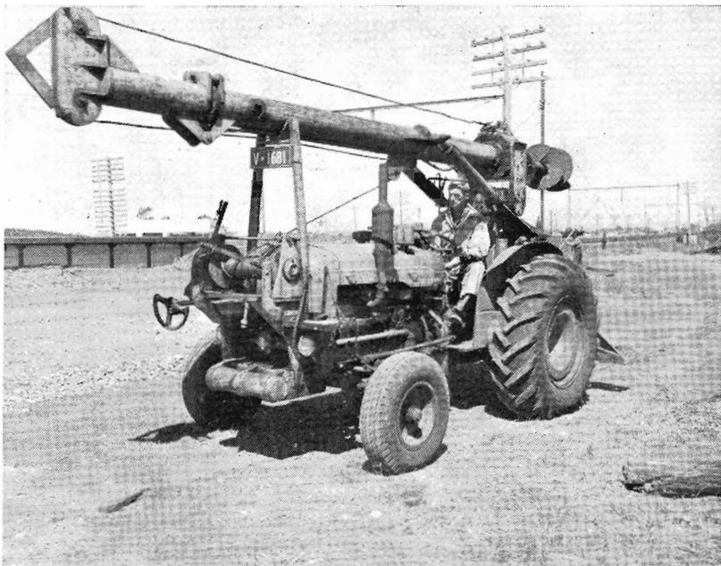
(Above) THIS machine is a combined earth borer and pole erector. As it here backs into position at St. Albans, the boring member is astride the petrol-driven vehicle. The driver mechanically tilts the borer—which has an interchangeable, rotating auger—to make the hole. After the machine hoists the pole, fixing is completed by manpower.
