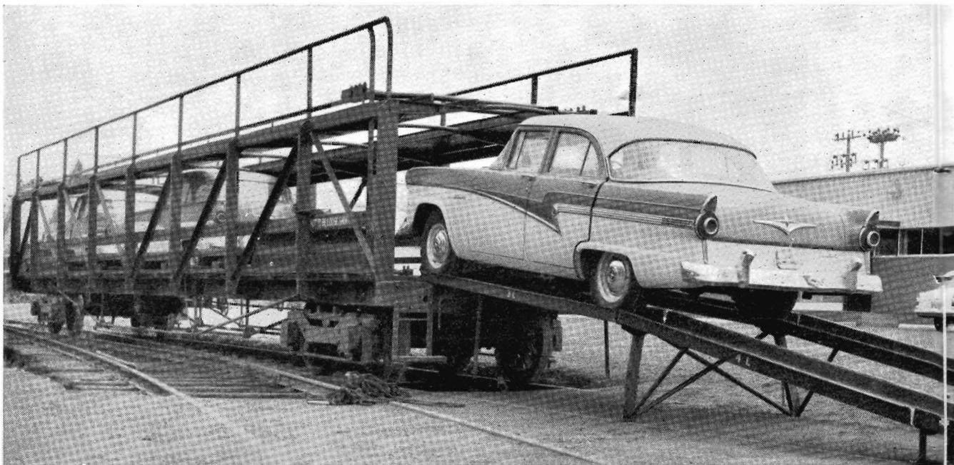
UNDER test at Ford Motor Company's Works, Geelong, was this new V.R. two-tier motor-car carrying rail wagon. Portable ramps were used for demonstration purposes; fully or semi-fixed ramps will be provided at loading and unloading points. Successful initial trip was on a recent Melbourne-Adelaide goods train.
