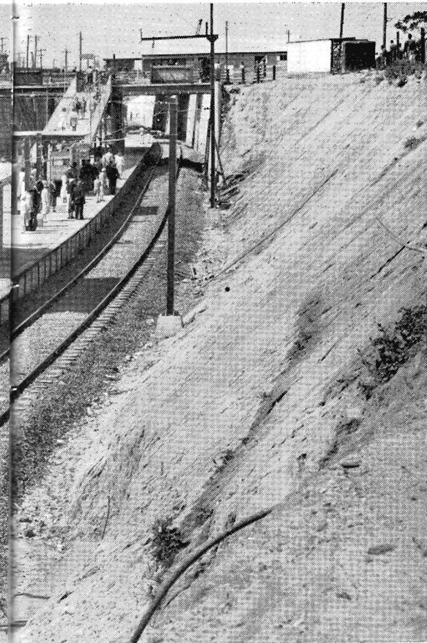
Excavation was made to a depth of 19 feet. At left of this picture a building was constructed to serve a "through" express track.
