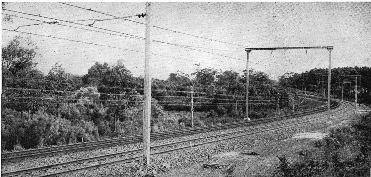
STRADDLING this fine stretch of the Gippsland electrified line are some of the "newer, simpler type of overhead masts enabling us to make a saving of £2,000 per mile".
