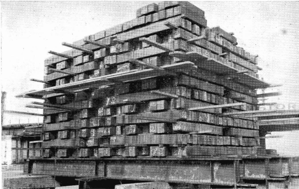
**WHAT'S THIS ?** Answer: three hundred tons of steel blooms, (for making railway axles), which were lent last month by the department to the builders of the King Street bridge across the River Yarra, Melbourne. Loaded on top of a concrete pile, this mass of steel was intended to simulate the ultimate stress to be carried when the bridge is finished.
