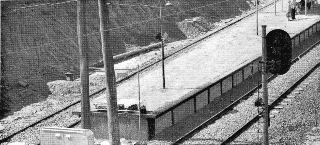
TAKING shape last month was the big grade separation and station re-building project at Moorabbin. Estimated cost of the grade separation at Nepean Highway and South Road is £437,000.
