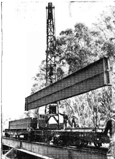
GIRDERS being swung into position for the standard gauge track over the Seven Creeks, Euroa.
