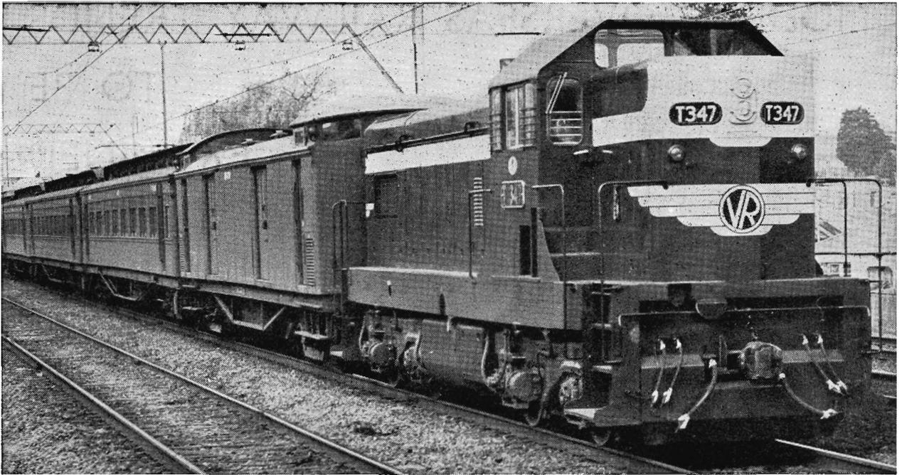
AT the head of this passenger train is a T class 900 h.p. dual-purpose diesel-electric (first of 10 now on order). It is additional to the 27 which started on the V.R. four years ago.
